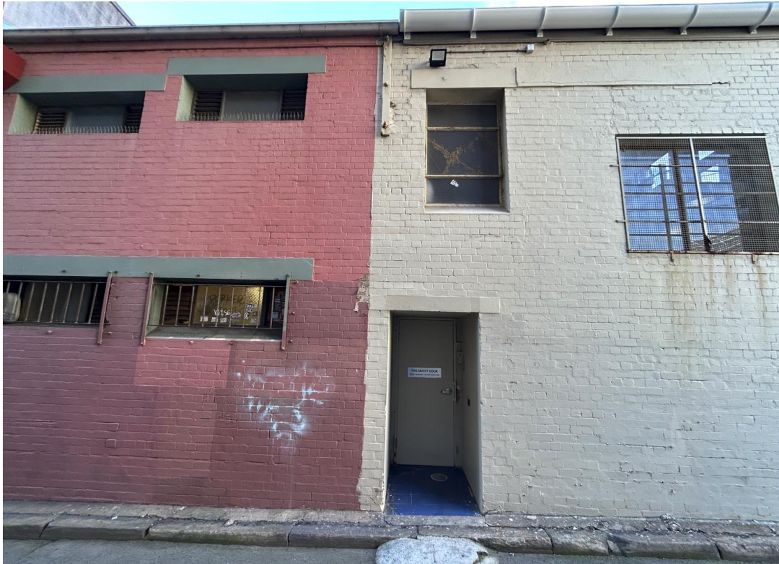
Figure 8: A fire exit to Grafton Lane which is accessed from the subject site and is located within the adjoining lot (1 Grafton Street, Chippendale)
