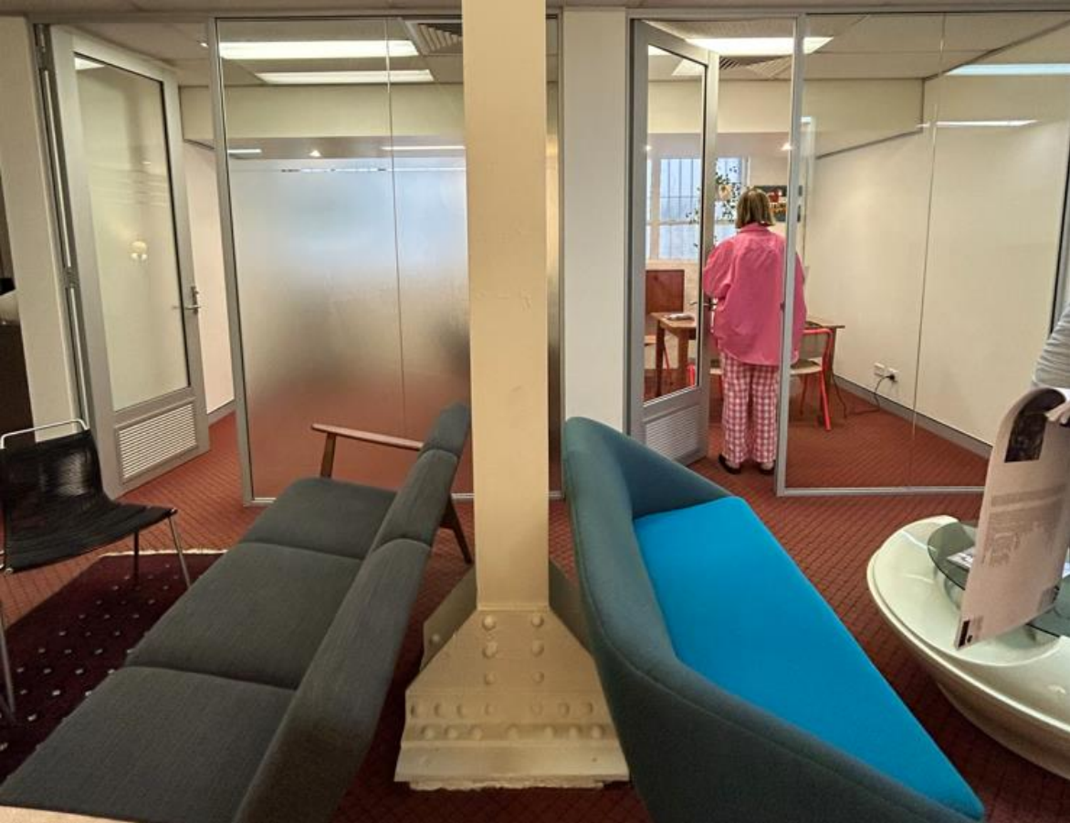
Figure 10: Interior with an example of a steel column to be retained
